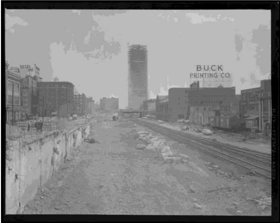
Figure 13 the Massachusetts Turnpike extension under construction. Kenmore Square is off-camera to the left. The Hotel Wadsworth is visible in the middle left. Newbury Street (left) hangs to the parallel edge of the canyon. The Prudential tower is under construction 19 Photo taken from Brookline Ave. Circa 1965. , Courtesy of the Boston Public Library, Leslie Jones Collection
