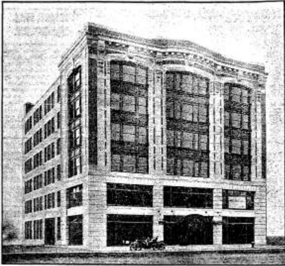
Figure 24 Peerless Motor Car Building, 1910
